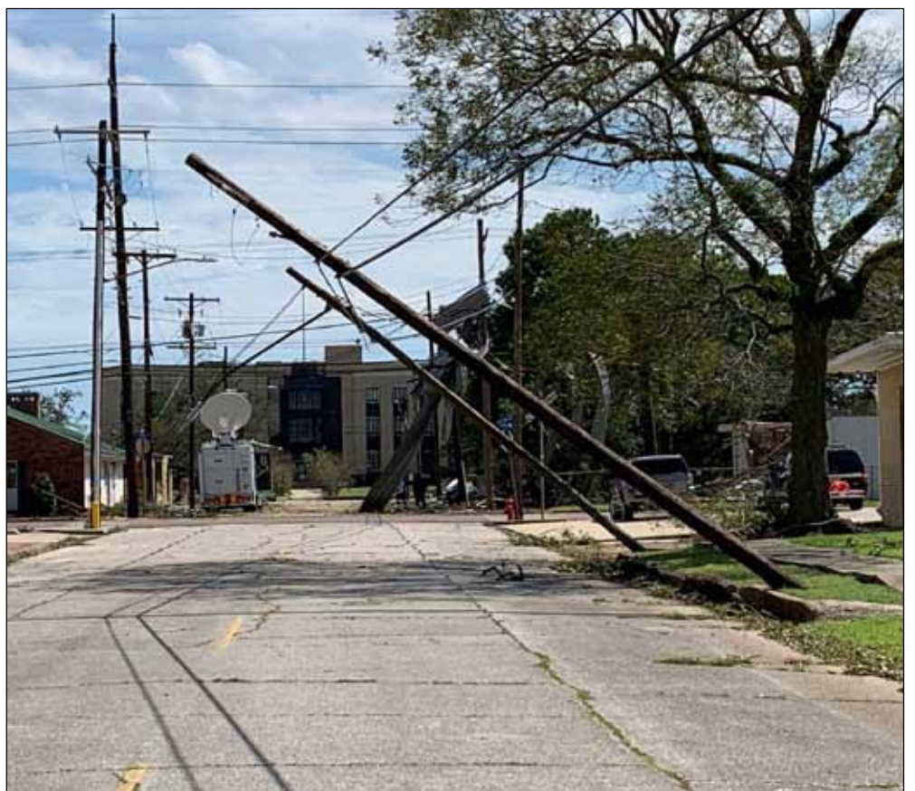
The look down 7th Street Thursday afternoon from Orange's old City Hall to the Orange County Courthouse was a bumpy one, highlighted by downed electric lines, bent over utility poles, a destroyed Stark Foundation warehouse and a damaged front of the courthouse. The white dish in the center is a television satellite truck supporting a crew doing remote broadcasting.
